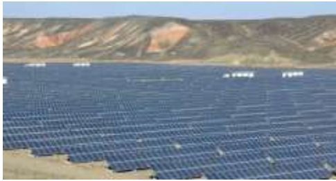
Fig.1. Photovoltaic power station
